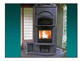
Site-built or site-assembled solid-fueled heating device, consisting of a firebox, a large masonry mass, and a maze of heat exchange channels. It stores heat from rapidly-burning fires within its masonry structure, and slowly releases the heat into the home throughout the day.
